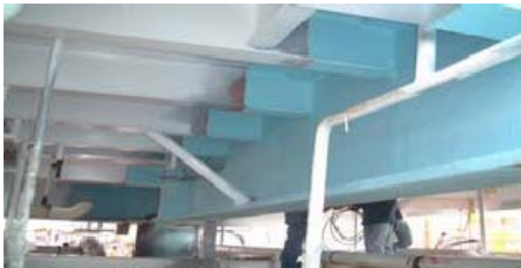
Typical Firetex M93 coatback scenario on underside of deck
